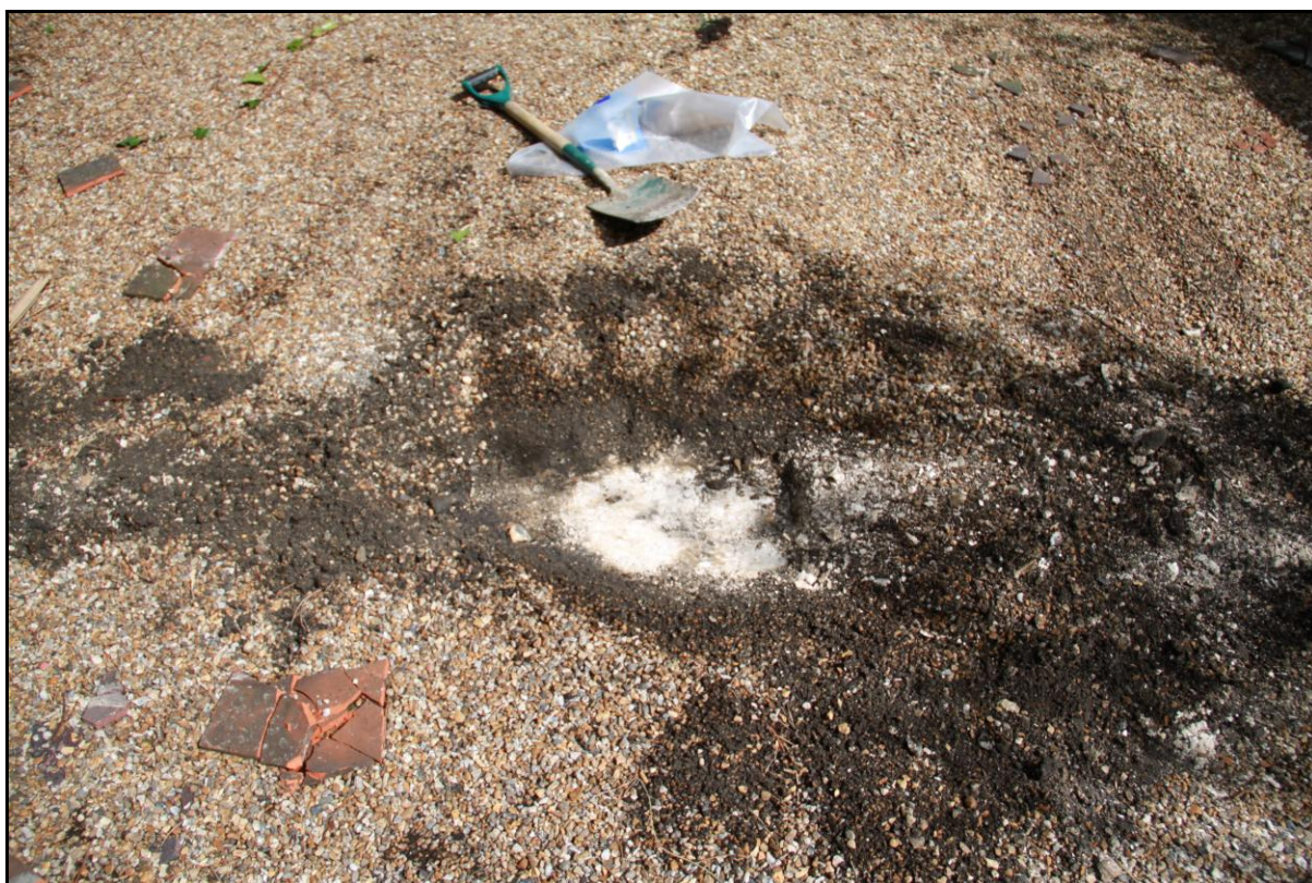
Fig. 4 Test pit on front drive
